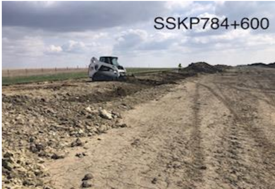
Sunken Access plug
