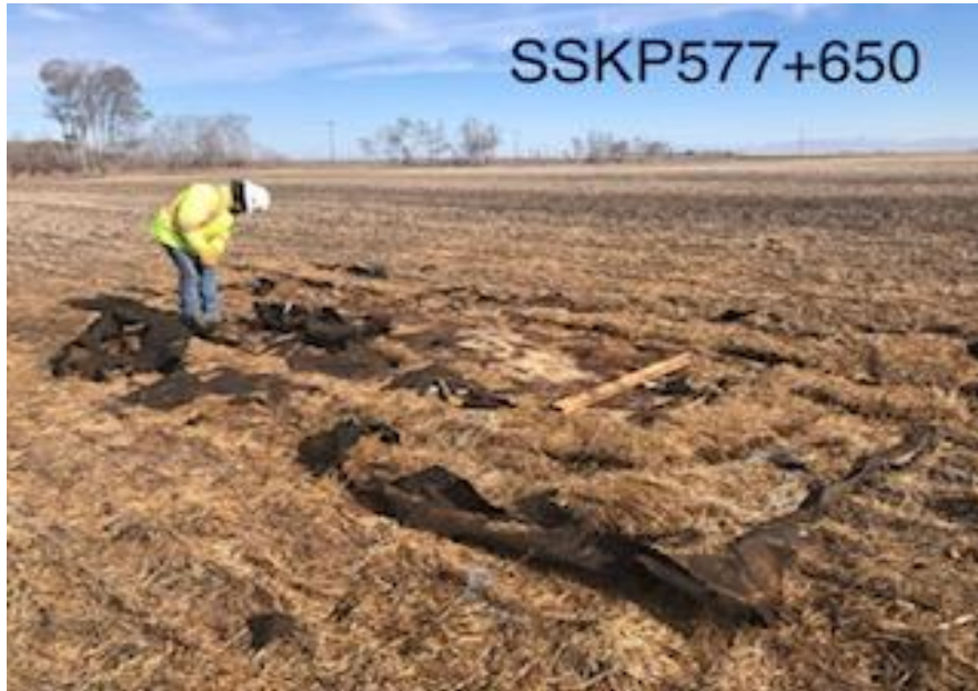
Filter bag being removed from dewatering site
