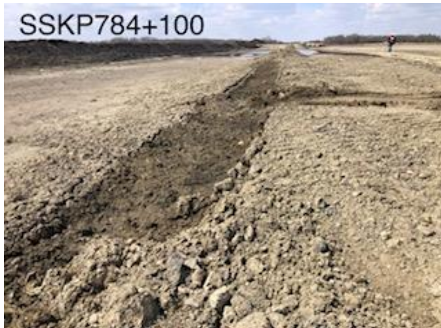
Working on access plug
