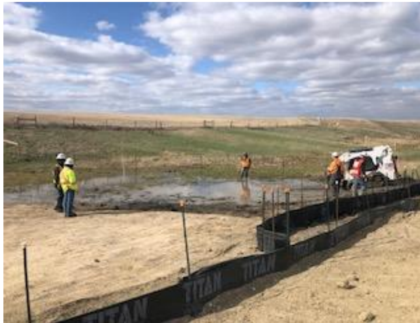
Kronau Creek sediment removal
