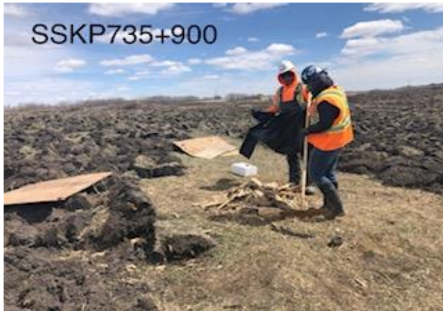
Debris being picked up at dewatering site
